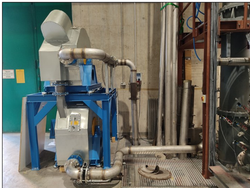
Figure 4a. Updates at the pilot plant. The in-series blowers are displayed in this photograph. These are key assets for the newly installed flue gas paths.
