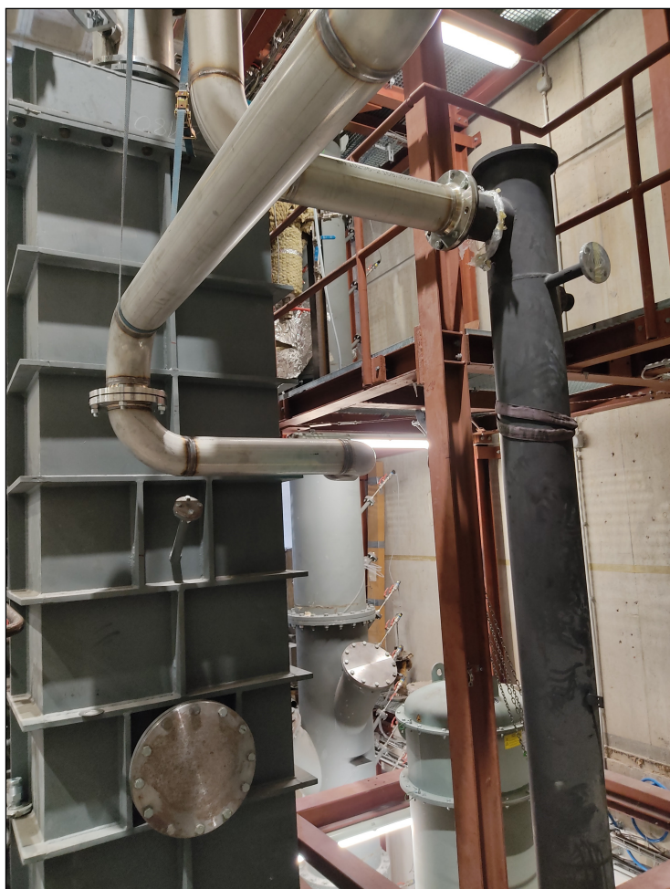
Figure 4b. Updates at the pilot plant. The photograph depicts a detail of the new flue gas path under construction. The new cooler and the filter can be seen.
